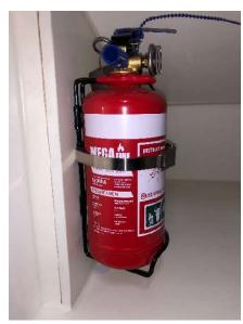
This fire extinguisher is a chemical powder perfect for putting out fires caused by electrical fault or liquid fuels.
