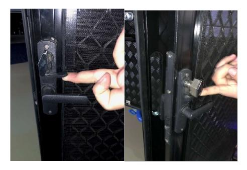
Lift the latch and the screen door will separate.
